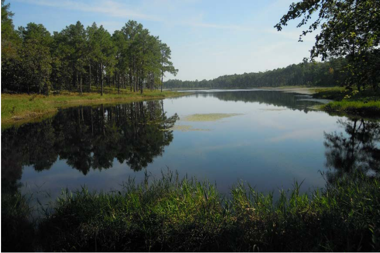
Figure 6. View of McKiethan Pond looking north from the crest of the dam.
