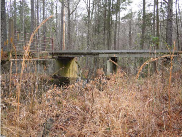
Figure 12. View of the upstream side of the spillway and vehicle bridge.
