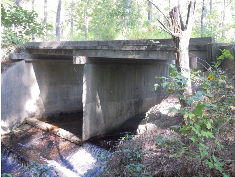
Figure 8. View of spillway looking west from the downstream bank.
